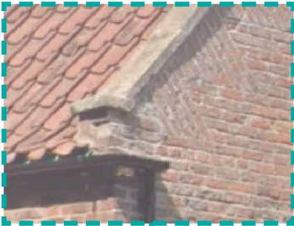
Stone coping gables Pantile roof
