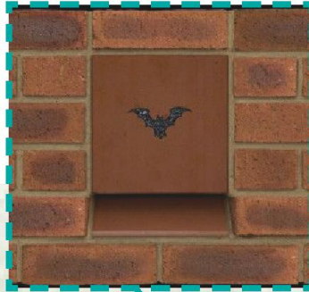
Built in bat boxes to side elevations
