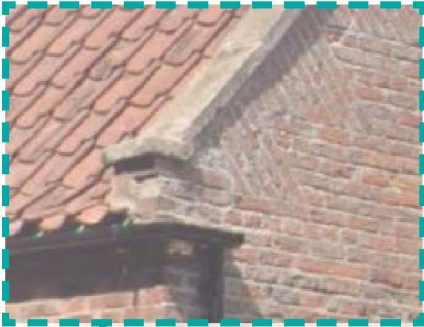
Brick detail to side elevations
